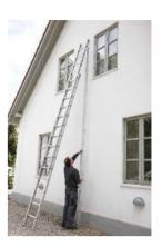
10. Drilling and rawlplugs (anchors) are put into the holes.
