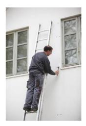
11. The ladder is installed again and the mounting screws are tightened. It is recommended to install the top bracket first and then continue down.
