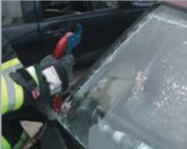
Glass saw for easy cut out of multi-layer safety glass
