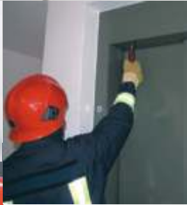
Key for emergency locking / de-locking of lifts
