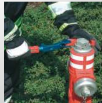
Servicing the spindle of the above-ground hydrant
